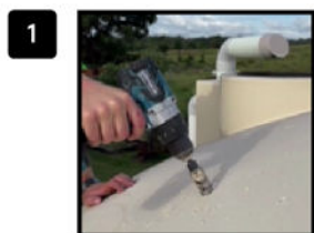
Drill hole above overflow level. Ensure the hole is clean, deburred and will not damage the cable.
